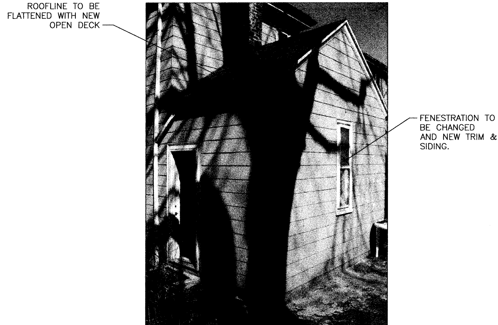
5 EXISTING SOUTH ELEVATION NTS
